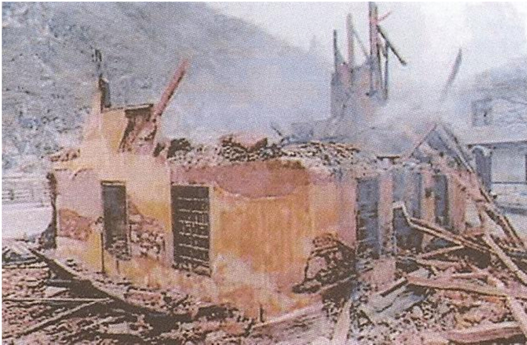
Photo 6. Albanian League of Prizren, burned and destroyed on March 27, 1999 (source: Shukriu, 2001)
